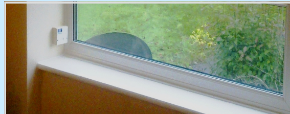
Full Renovation required, both wood sealant & primer + mould biocide. Finished sill with 2 Coats Dulux Gloss
