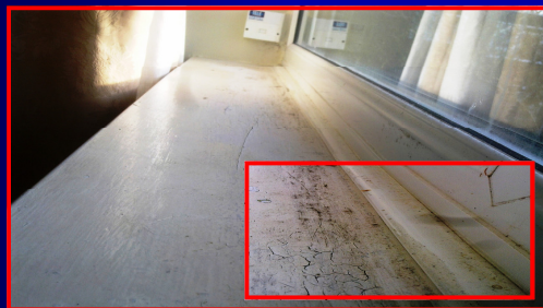
Windowsill condensation damage Mould in Alcove painted plaster Damp rot around fixing nail
