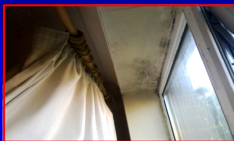
Windowsill condensation damage Mould in Alcove painted plaster Damp rot around fixing nail
