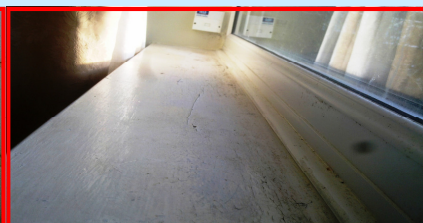
Full Renovation required, both wood sealant & primer + mould biocide. Finished sill with 2 Coats Dulux Gloss
