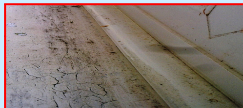
Full Renovation required, both wood sealant & primer + mould biocide. Finished sill with 2 Coats Dulux Gloss
