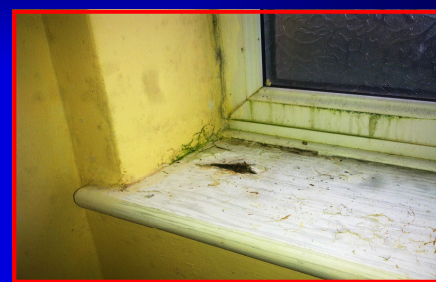
Windowsill condensation damage Mould in Alcove painted plaster Damp rot around fixing nail
